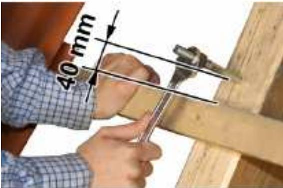
6a: Leave the roof free of tiles (1260mm for one panel), then mount the coach-bolts and rails as described in step 1.
